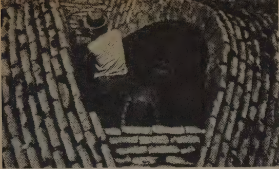
Constructing a vault for a skylight.
